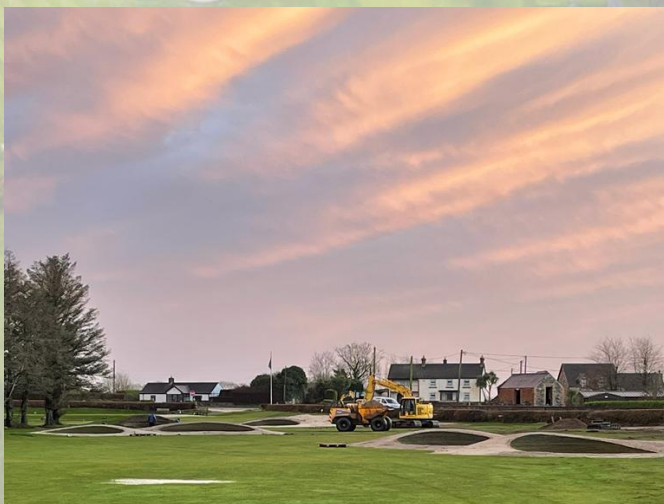
View of the new bunkers on the 9 th hole
